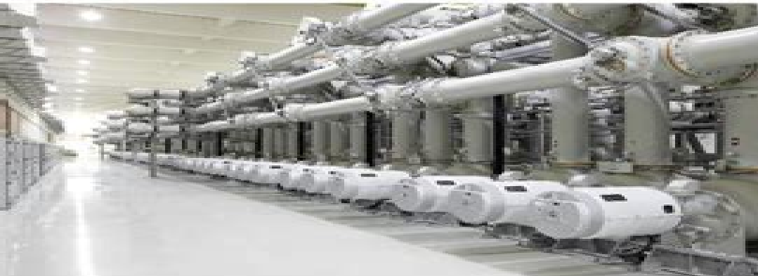
Gas-insulated Switchgear
