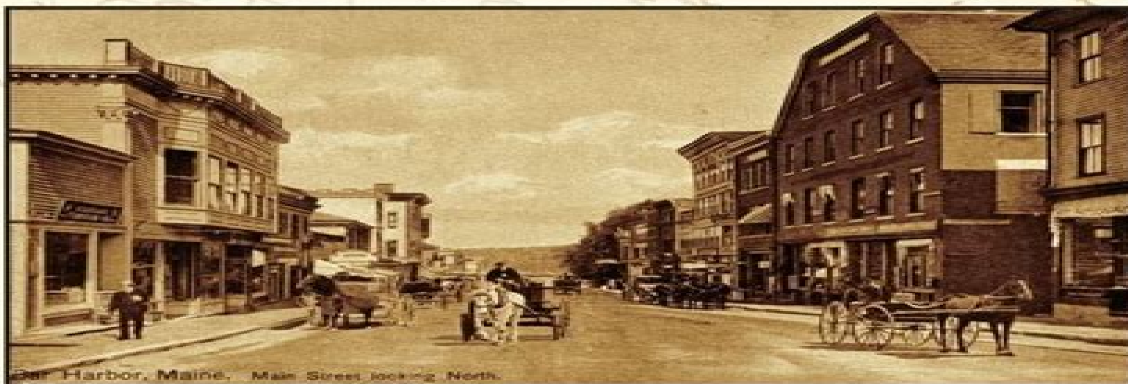
Bar Harbor, Maine. Main Street looking North.
