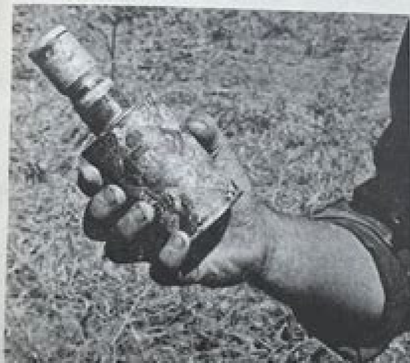
Figure 2.--Shown is a VC grenade made from locally available materials including a carelessly discarded "Coke" can.
